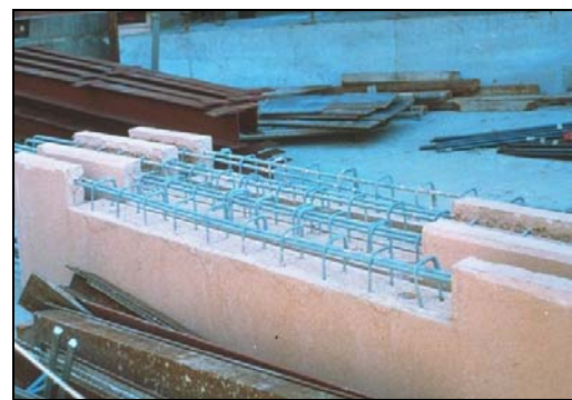
Spandrel beams
