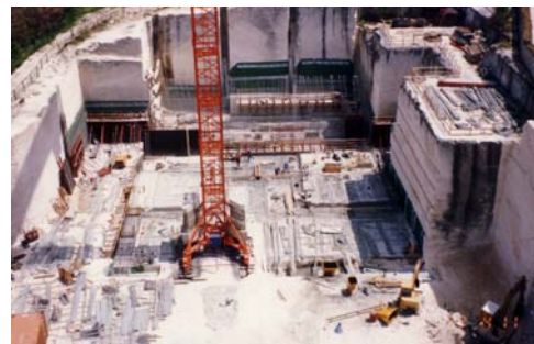
d) Tynes Bay waste-to-energy plant foundations with 100% galvanized reinforcement.
